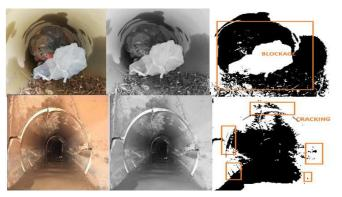
Fig. 7. Image Processing Sewer Defect Analysis.
