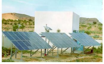
Fig. 10. The Photo of the PV Pumping System Installed in Louata-Tunisia.
