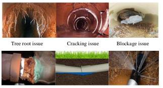
Corrosion & Bellied pipeline issue Leakage issue Deterioration
