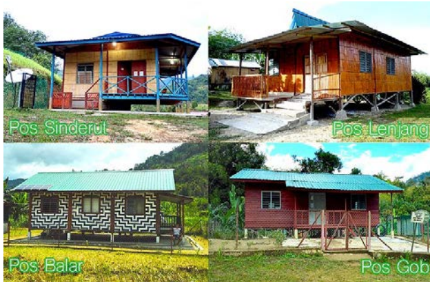
Fig. 3. The Four unique TPOA Telecentre Buildings.
