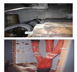
Fig. 2. Apparition of the dew inside the electric cells
