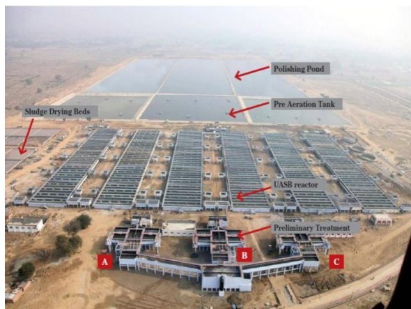
Fig. 1. Aerial Photograph of Bharwara WWTP.
