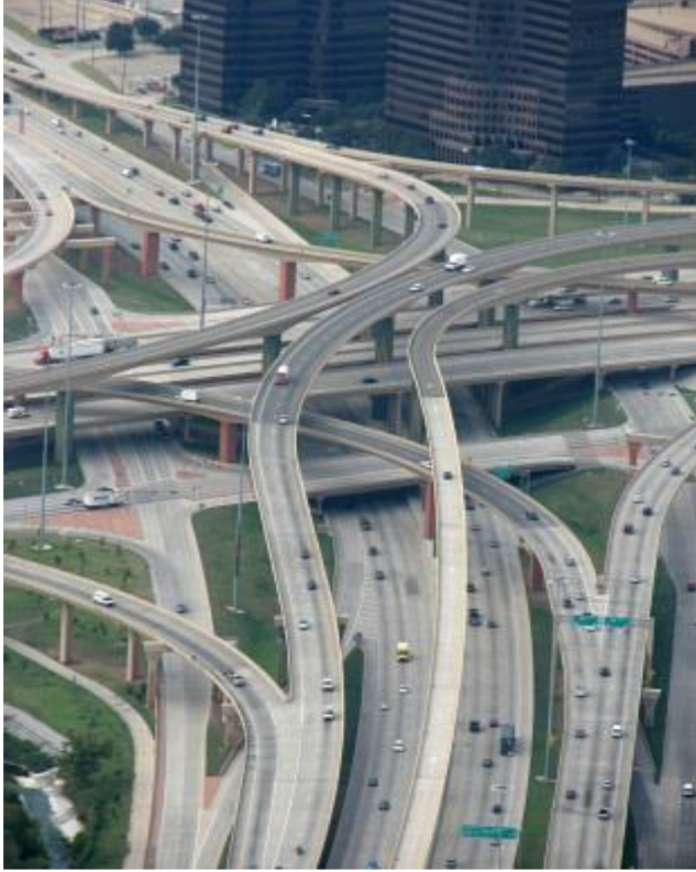
Fig. 5: A five-level interchange (The High Five Interchange in Dallas, Texas, United States).
